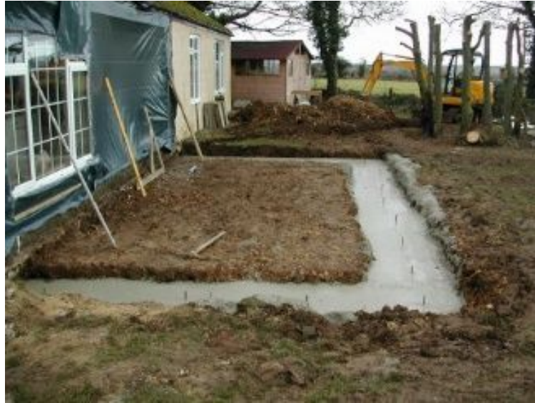
Laying the foundation
